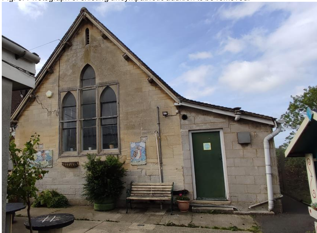
Fig. 8: Photograph of existing unsympathetic addition to be removed.
